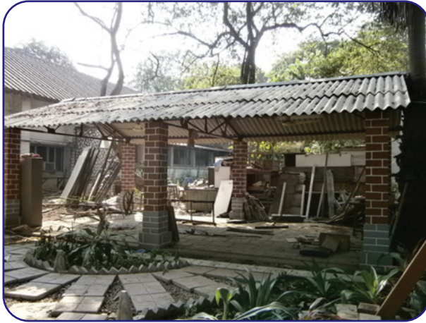
Pilot structure constructed inside IIT Bombay campus completely using the eco bricks
